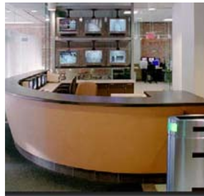
24/7/365 Security personal Card Access with Recorded CCTV
